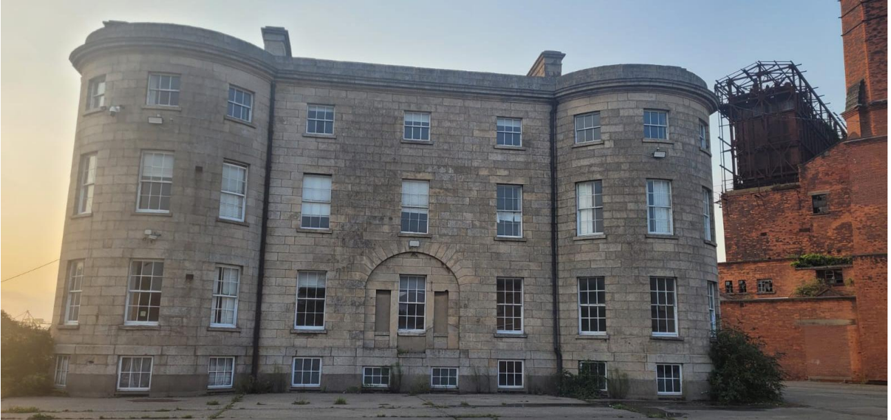
Plate 2: Building 2 – Modern sheds adjacent to Building 1, Poolbeg, Co. Dublin.
