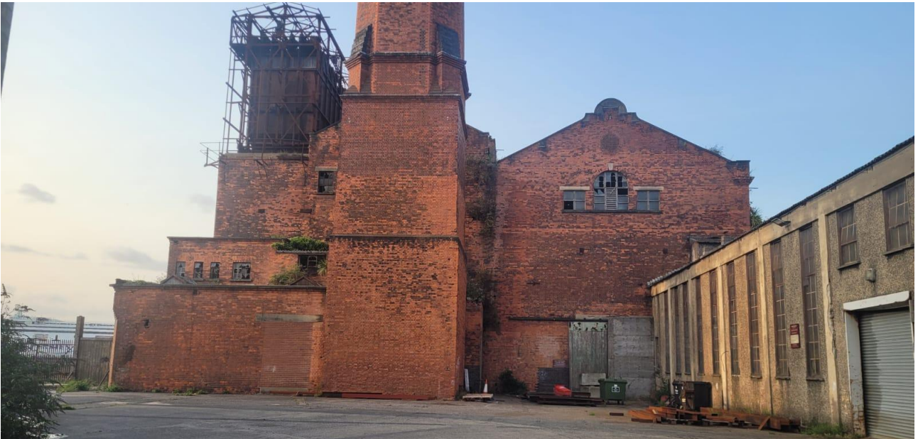
Plate 1b: Building 1 – gable of main structure with section of Building 3 shown, Poolbeg, Co. Dublin.
