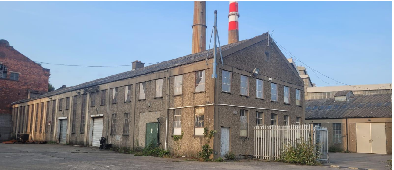
Plate 3: Building 3 – Modern sheds adjacent to Building 1, Poolbeg, Co. Dublin.
