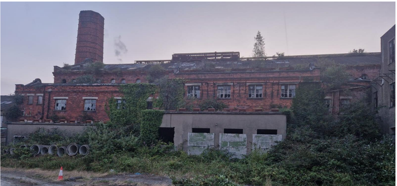
Plate 1c: Building 1 – rear of main structure of Building 1, Poolbeg, Co. Dublin.
